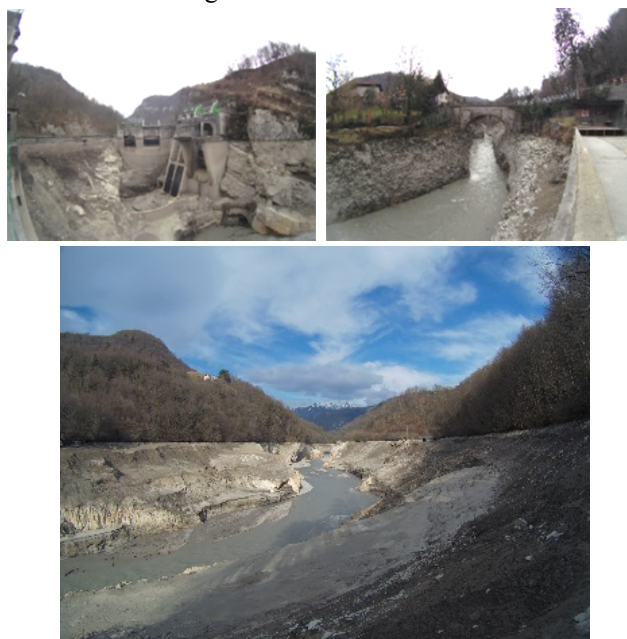
Figure 3. Emptied drains and banks.
